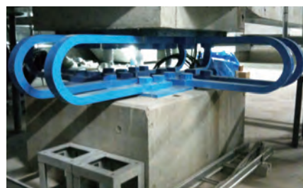
U型鋼材ダンパー U-shaped steel dampers
